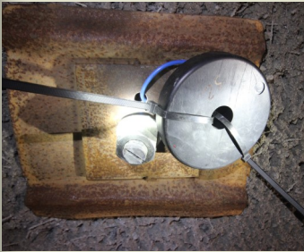
Radio donut cable tied to collar plate
